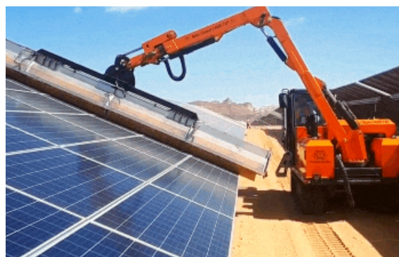
LAVAGGIO PANNELLI SOLARI SOLAR PANEL WASHING
